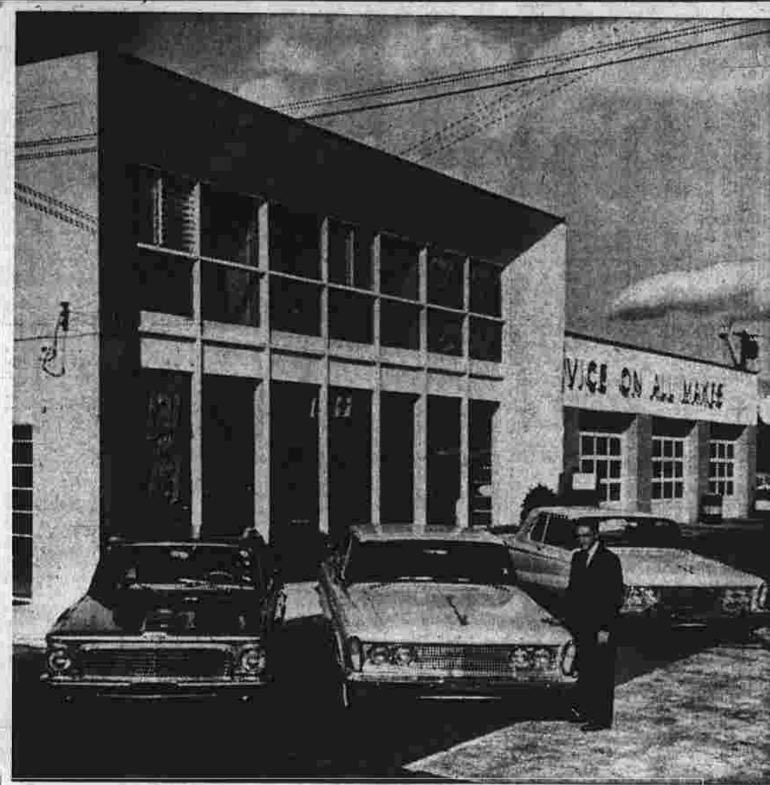
Manchester Plymouth Inc., Rt. 83, Talcottville, shows its new look on the recently remodeled and repainted facade. The former one-story building has lost its high ceiling show room which now houses company offices above the new car display area. The firm, under the ownership of Reuben Cutler (above), Joseph Kovalsky, and Lester Resnick, has been in business at the Talcottville site for two years. (Herald photo by Sateris).
